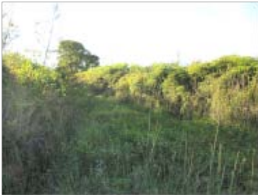
Constructed drainage channel ('Industrial Estate drain') traversing the beach ridge plain between Belongil Fields and Melaleuca Drive
