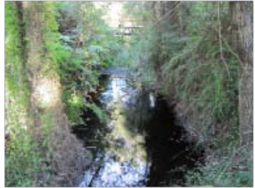
Constructed drainage channel ('Industrial Estate drain') traversing the beach ridge plain within southern section of Belongil Fields
